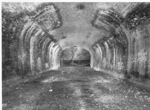
Looking north out of Bourne Park tunnel in March 2012.
